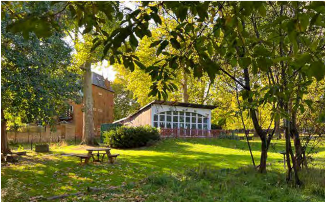
Image 4– Existing Bandstand Building
